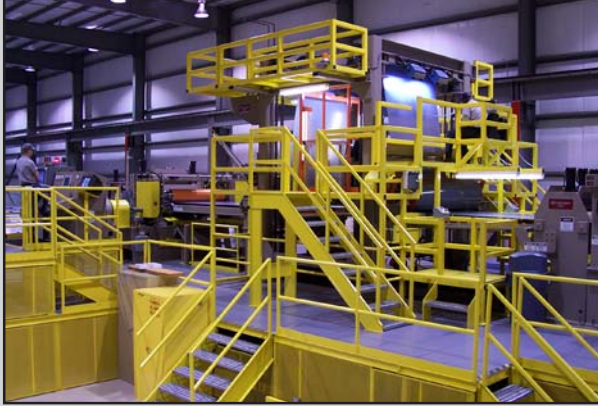
Top & Bottom Surface Inspection Tower
