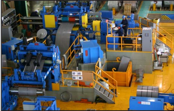
Exit end view. Notice the clear sight lines from the main operator station.
