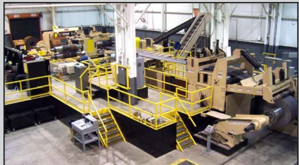
80,000# x 72" x 3/8" Slitting Line Exit End View
